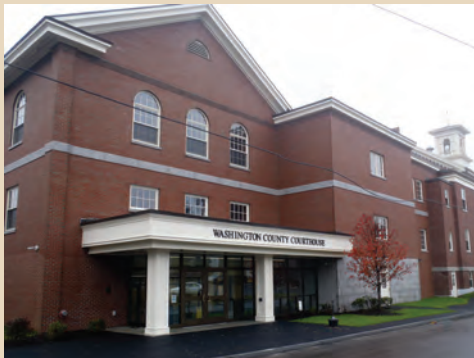
The Washington County Courthouse in Machias renovations and new addition, including the clerks' office, two new courtrooms, judicial chambers, a large conference room, and attorney-client conference rooms, were completed in July 2015.
